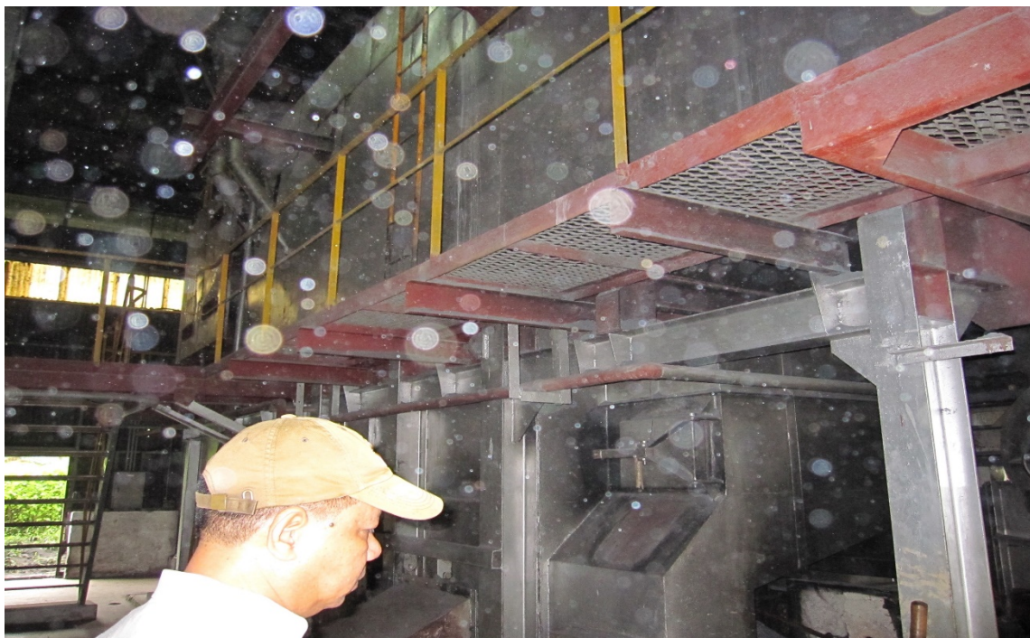
Fig. 7-2. Village in Myanmar supplied with electricity by rice husk boiler
